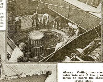
Coiling deep - sea Above: Coiling deep - sea cable into one of the great tanks on board the cablelaying ship.
